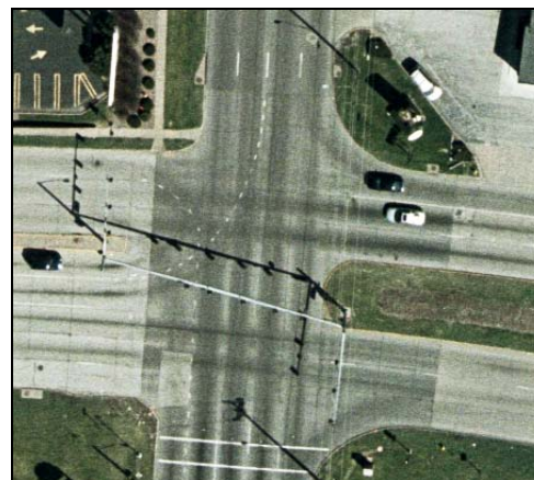
Figure 95. Kimberly Rd. & Brady St. aerial view.
