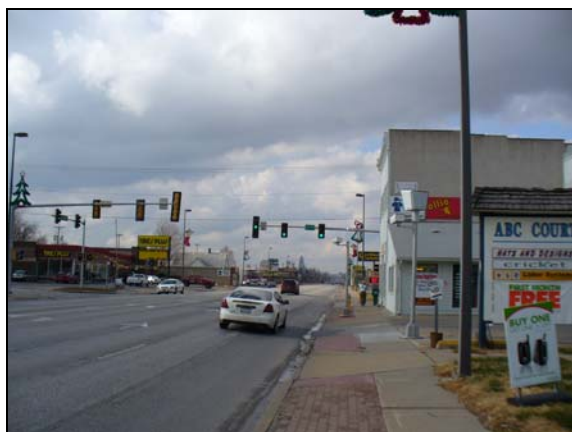
Figure 75. Broadway and 21st St. (westbound).
