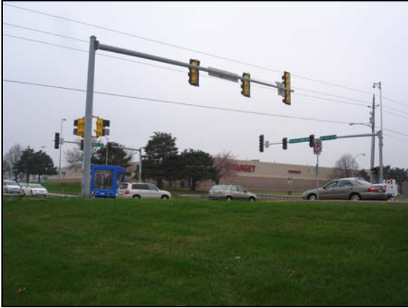
Figure 37. 35th St. & University Ave. (southbound).
