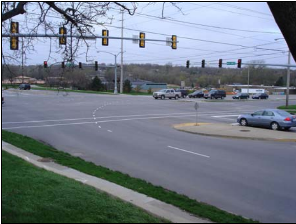
Figure 34. 86th St. & Douglas Ave. (southbound).
